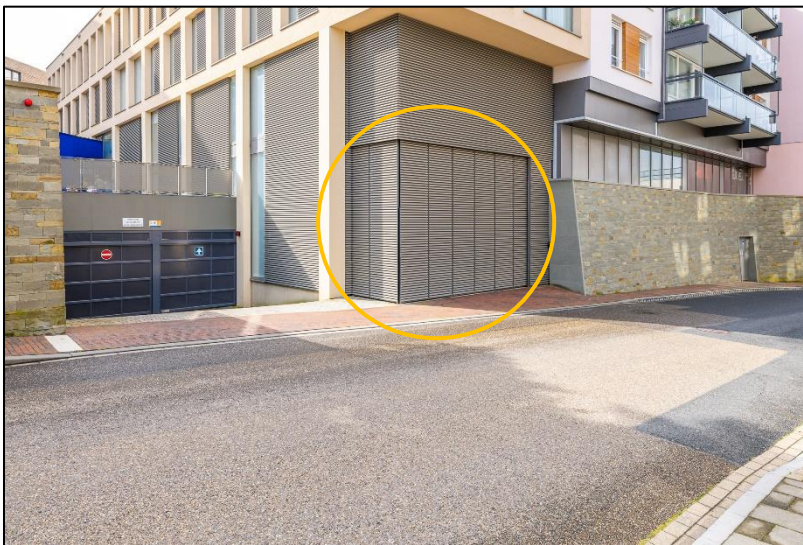
Entrance loading dock at the Mozartstraat at house number 5
